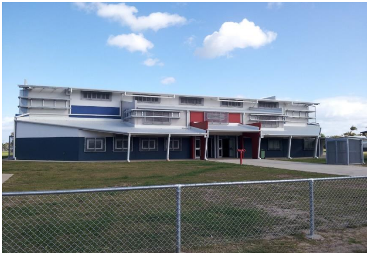
The Whitsunday Regional Council cyclone shelter, in the grounds of Proserpine State High School, Proserpine. A finalised Cyclone Shelter sub-plan is anticipated in February 2016 to replace the interim plans currently in existence.
