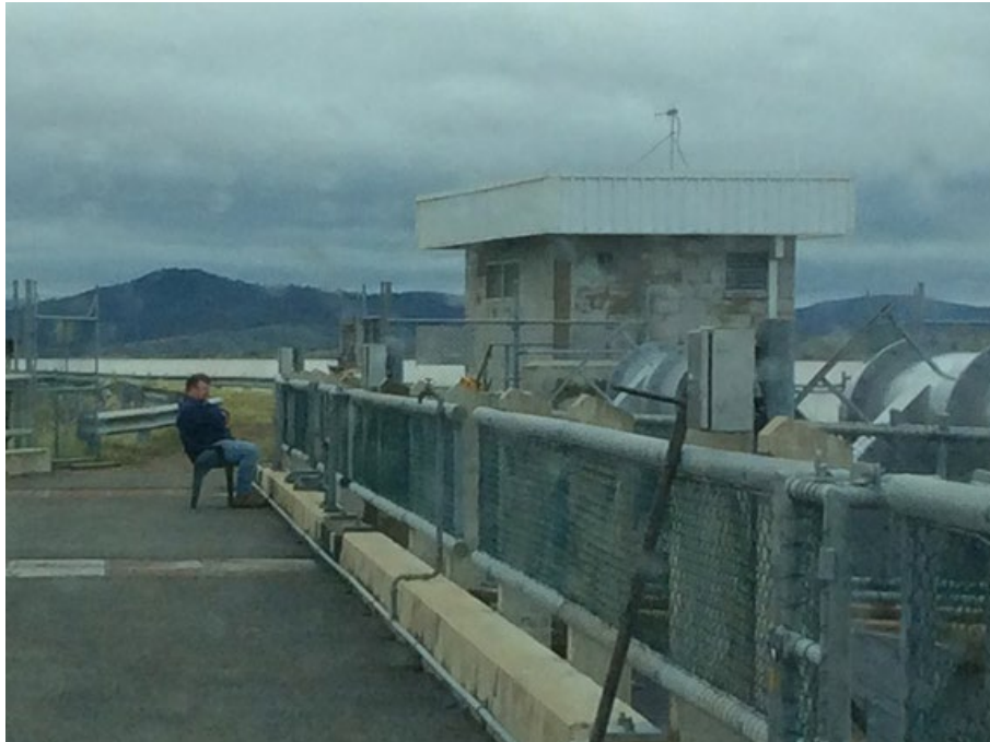
Right: Manual monitoring of the Callide Dam. SunWater, 2015
