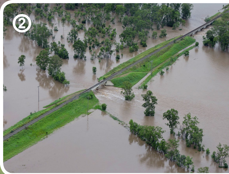
Below: Burnett Highway, rail overpass. Banana Shire Council
