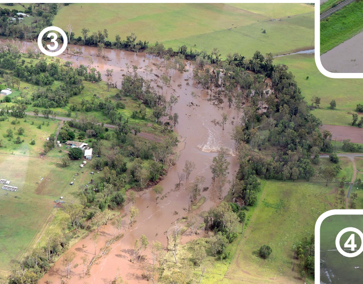
Above: Linkes Road, Callide Creek. Banana Shire Council
