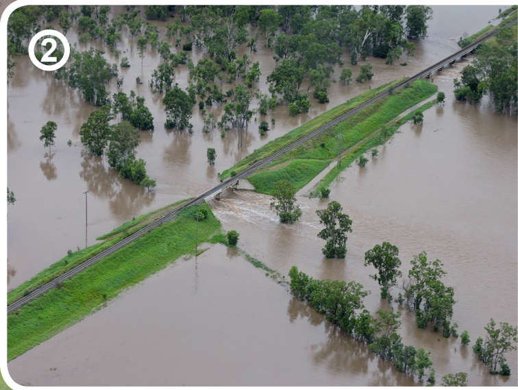
Below: Burnett Highway, rail overpass. Banana Shire Council
