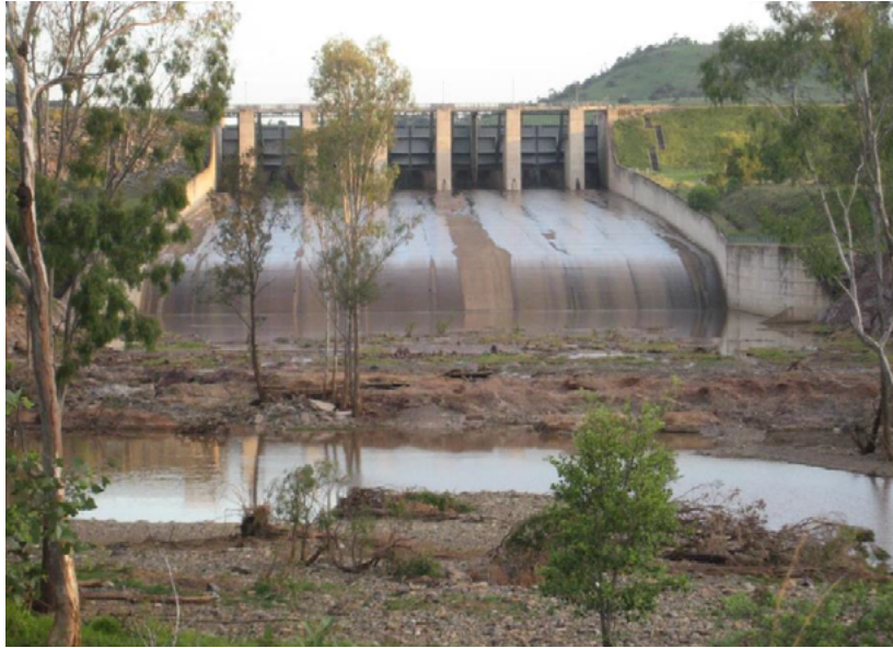
Figure 1-5 Callide Dam spillway following 2013 event (source: Water Solutions, 2013)
