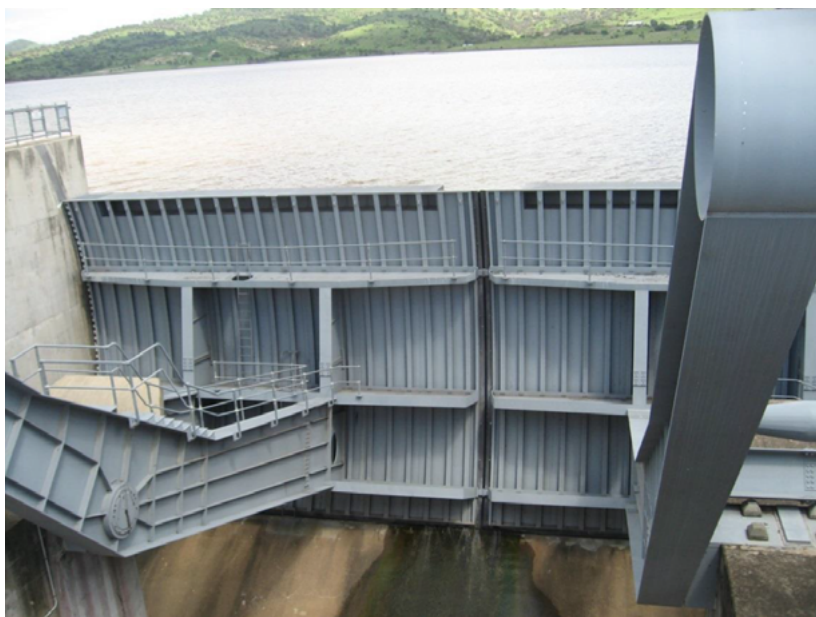
Figure 1-6 Callide Dam gates (source: Water Solutions, 2013)
