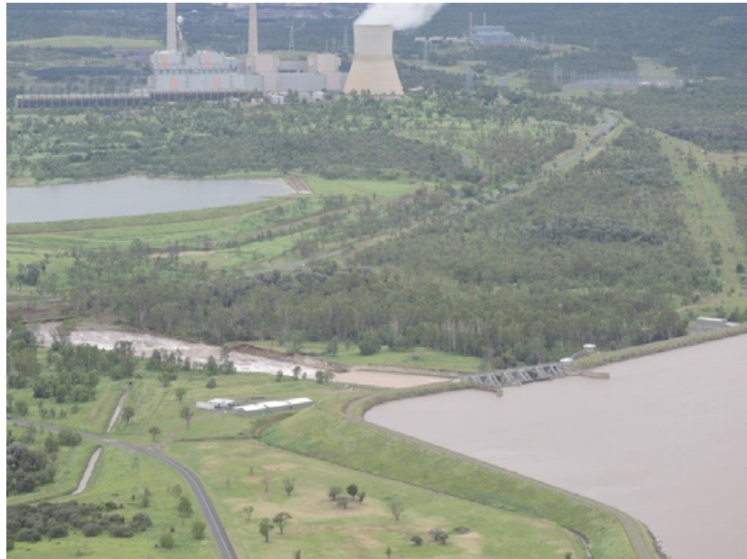
Figure 1-4 Callide Dam wall and gates, with Callide Power Station in background (source: Banana Shire Council)
