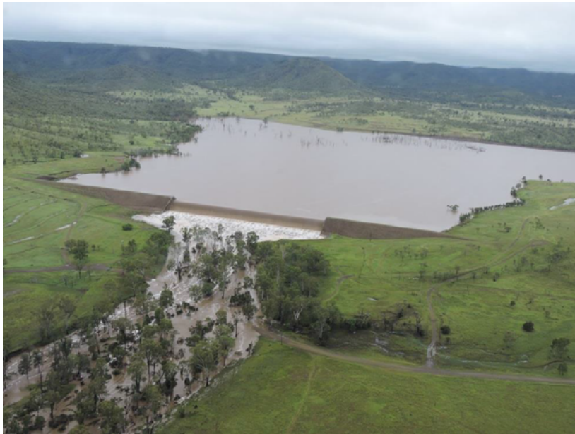
Figure 1-3 Kroombit Dam at 08:46 on 21 February 2015 (source Banana Shire Council)
